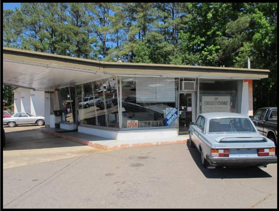
Figure 93: Phillips 66 Service Station, Office Section, Looking Northwest.
