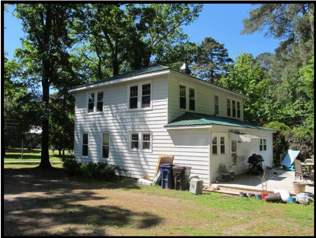
Figure 47: Buffalo Presbyterian Church Manse, Looking Southwest.
