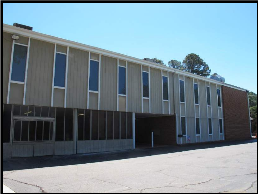
Figure 82: Elks Lodge #1679, Detail of Fenestration on West Elevation.
