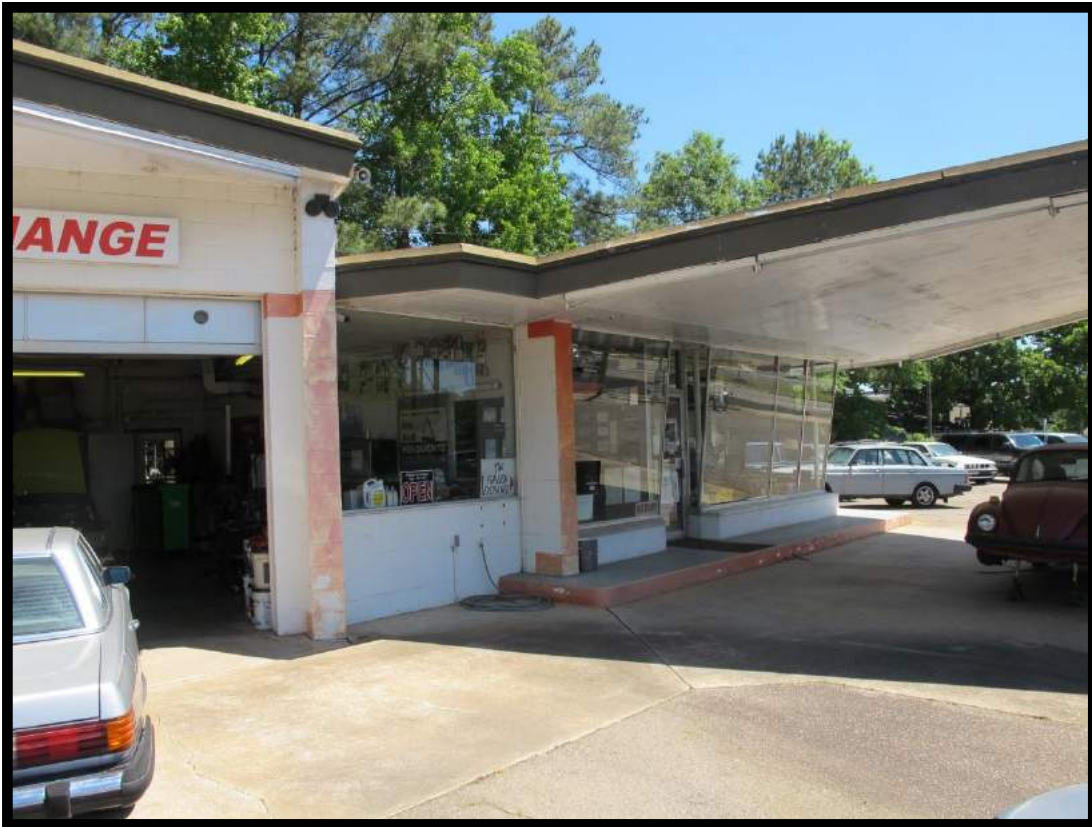
Figure 94: Phillips 66 Service Station, Connection Between Garage and Office Looking Northeast.
