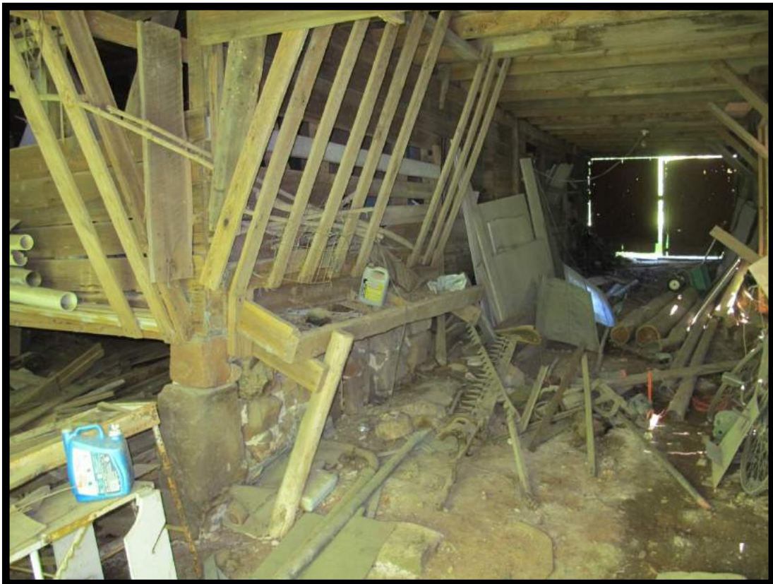
Figure 72: Arthur McIver House, Barn, Interior View of Drive-Through.
