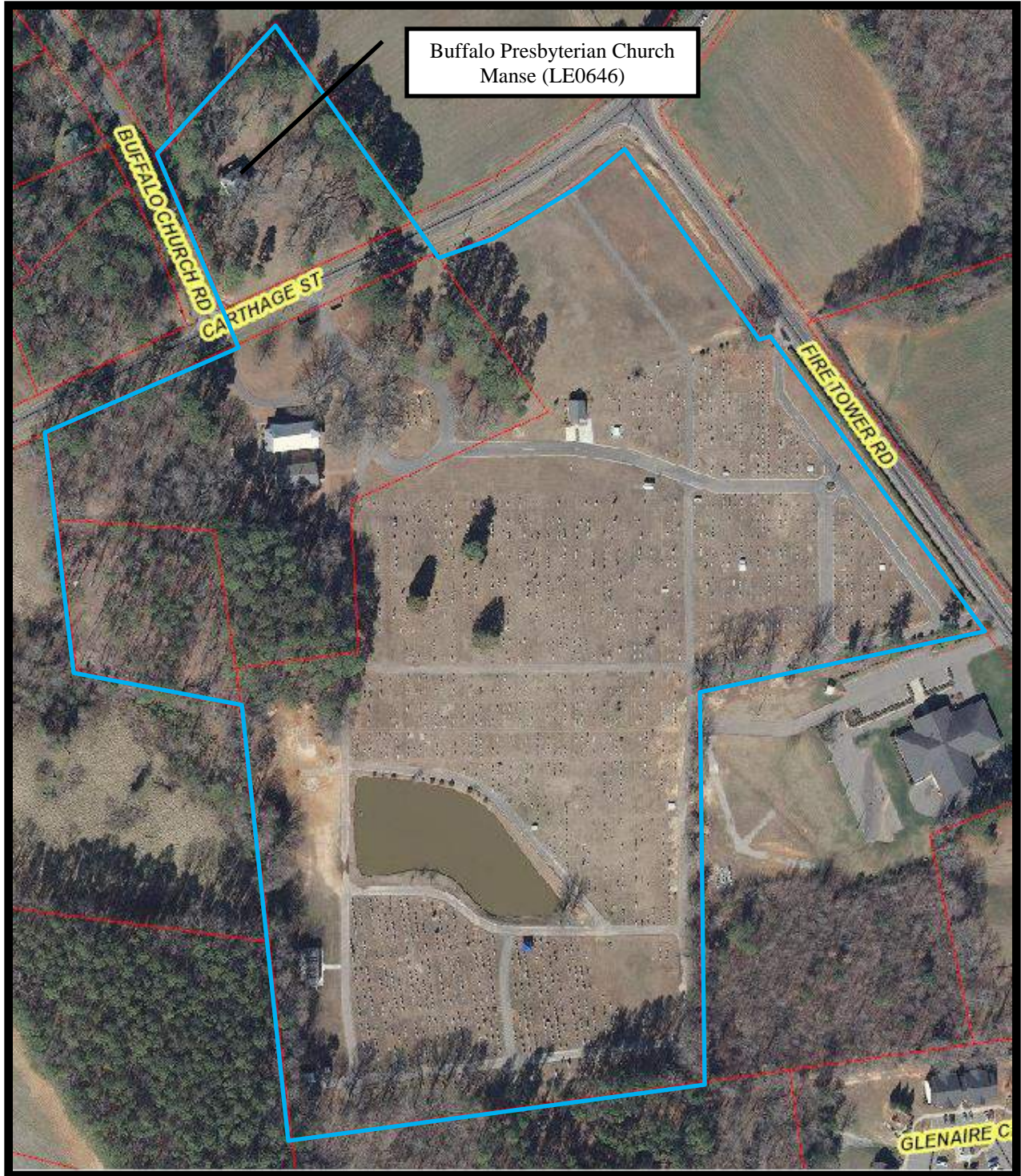
Figure 43: Aerial Map of Buffalo Presbyterian Church and Cemeteries, Showing the NRHP Boundary
