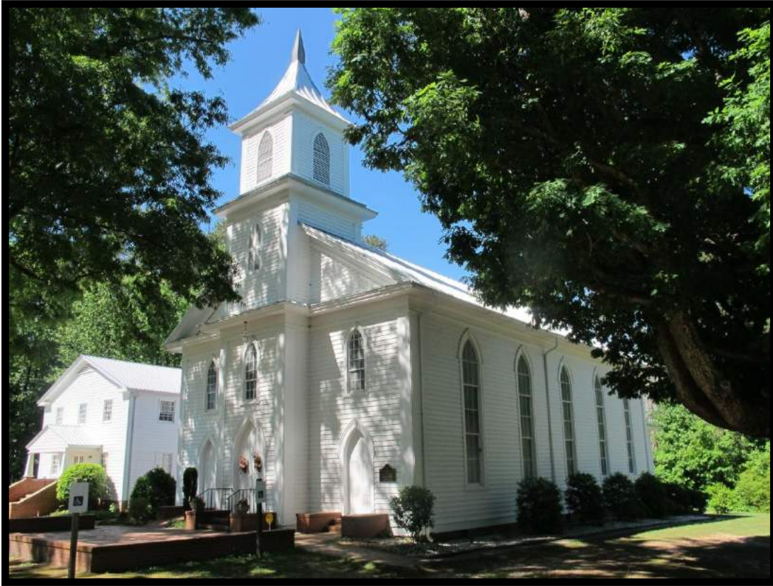
Figure 26: Buffalo Presbyterian Church, Looking Southwest.
