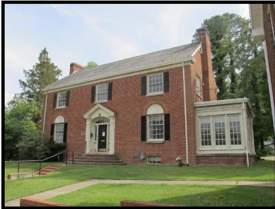
Figure 74: H. F. Ohler House, Looking Southeast.
