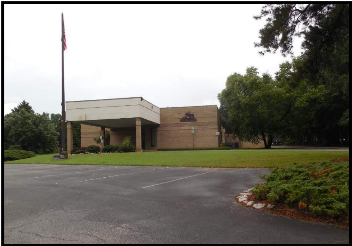
Figure 89: Elks Lodge #840 (Wilson), Looking Southeast
