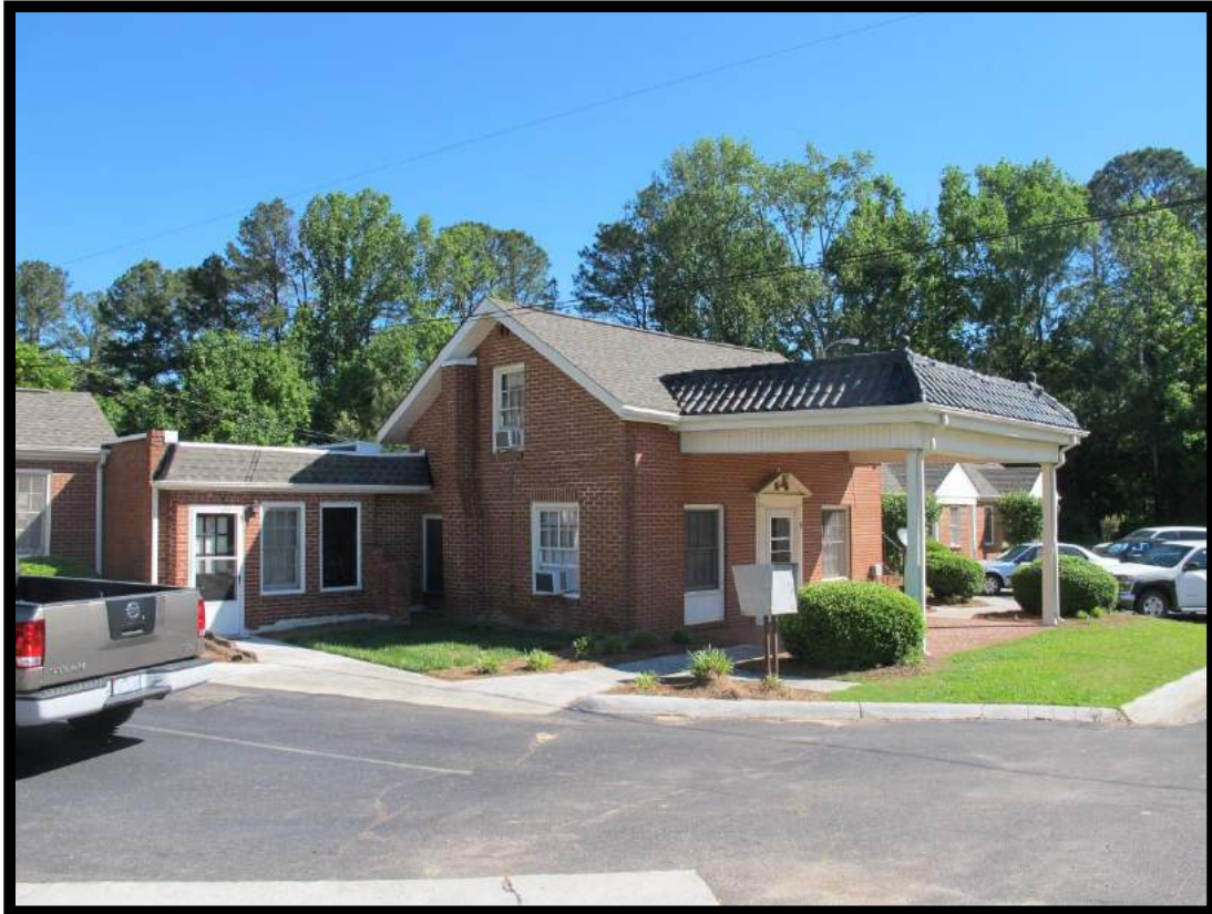
Figure 8: Jefferson Motel, View of Central Section and Flat-roofed Wing Looking North.
