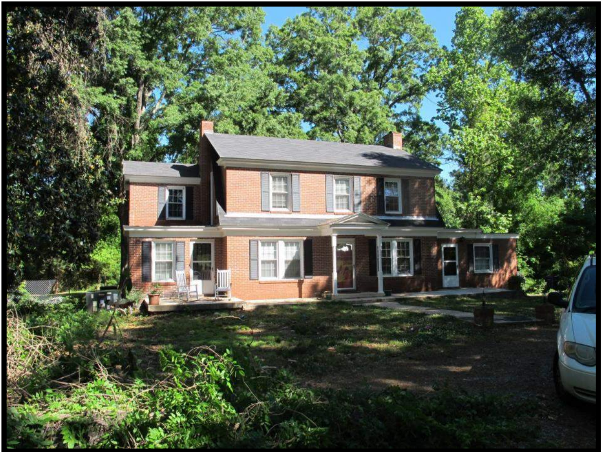
Figure 14: View of House Looking North.
