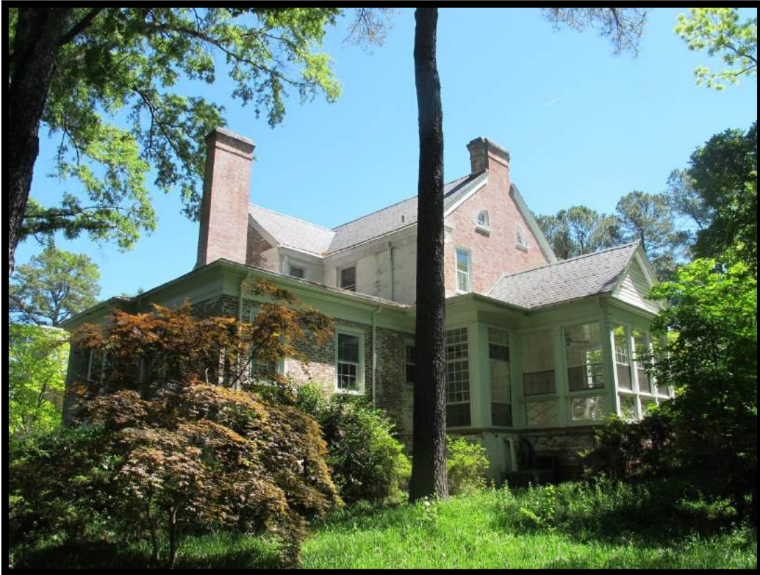
Figure 65: Arthur McIver House, Looking Northeast.
