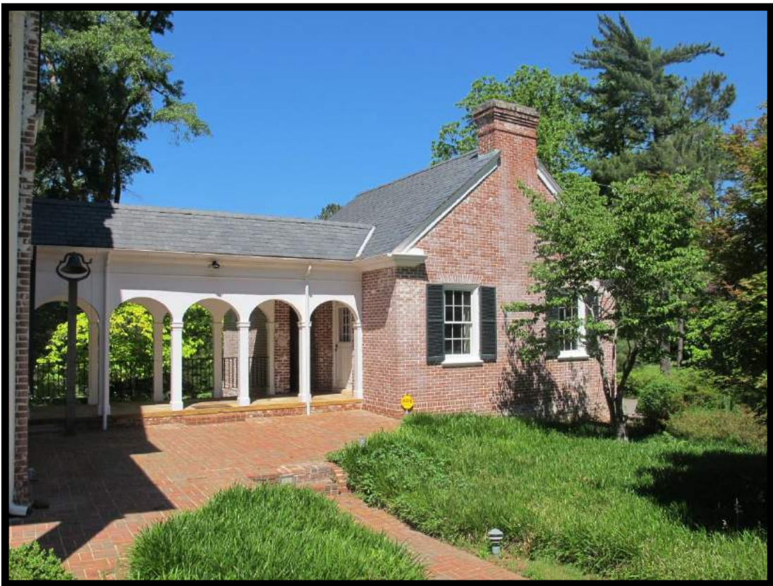
Figure 67: Arthur McIver House, Garage Looking Northwest.
