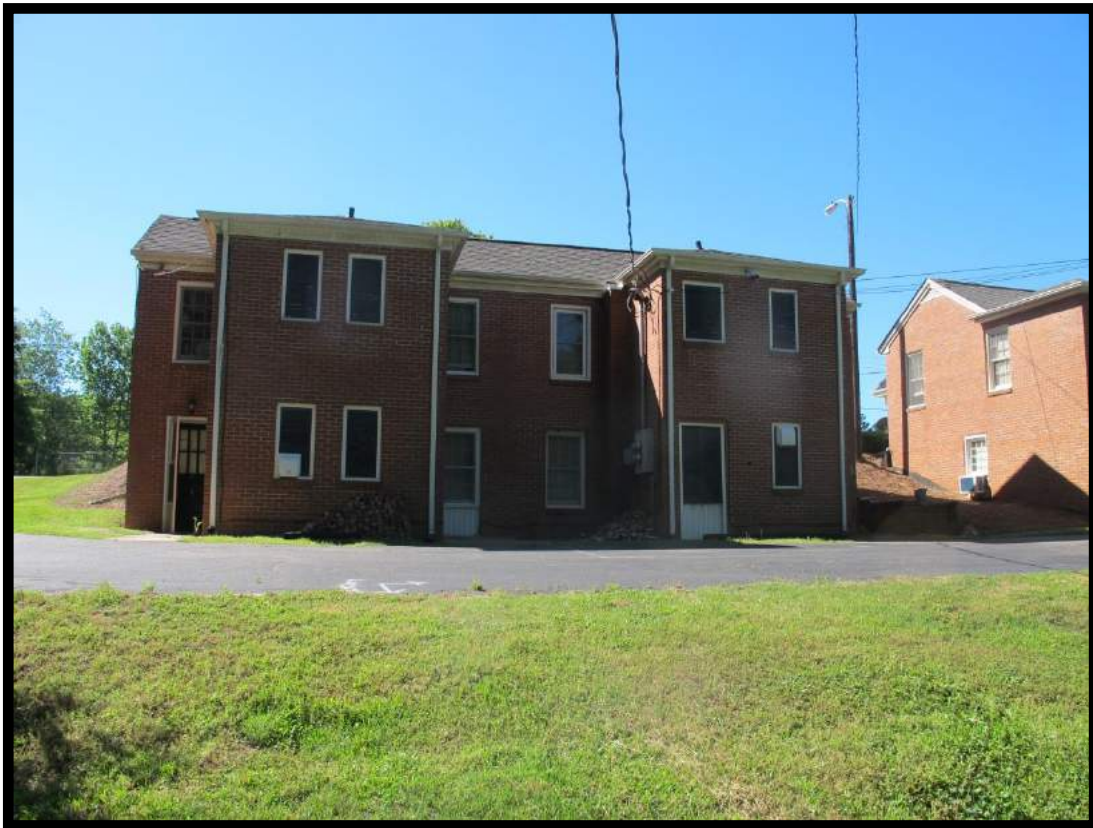
Figure 13: Jefferson Motel, View of Stand-alone Section Looking South.
