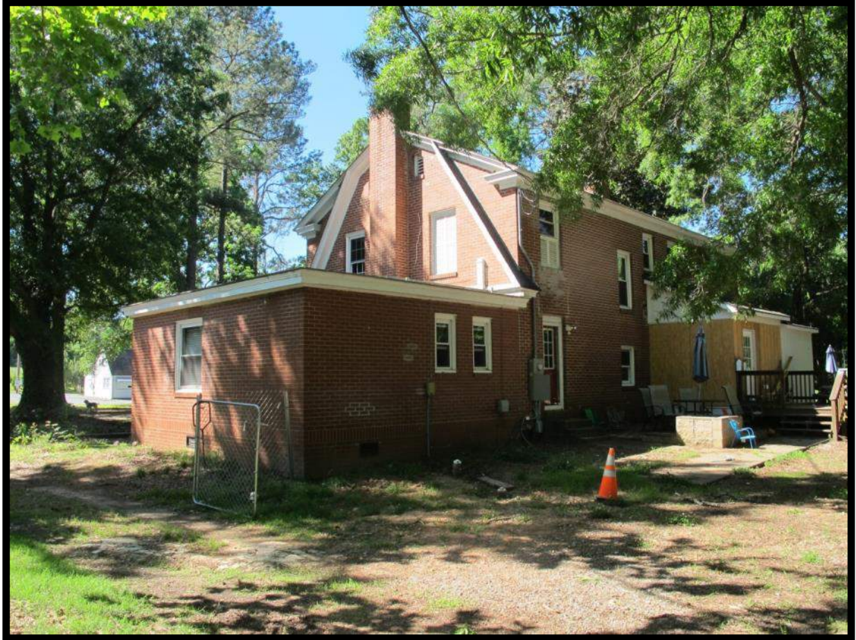
Figure 15: View of House Looking South.
