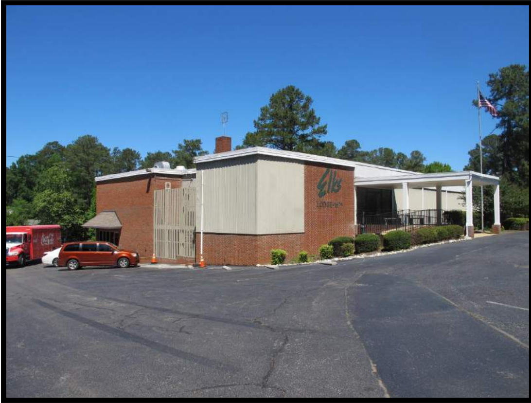
Figure 79: Elks Lodge #1679, Looking Northwest.
