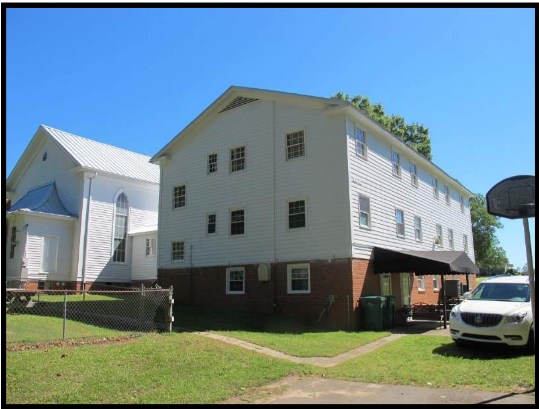
Figure 29: Buffalo Presbyterian Church, Educational Building Looking Northeast.
