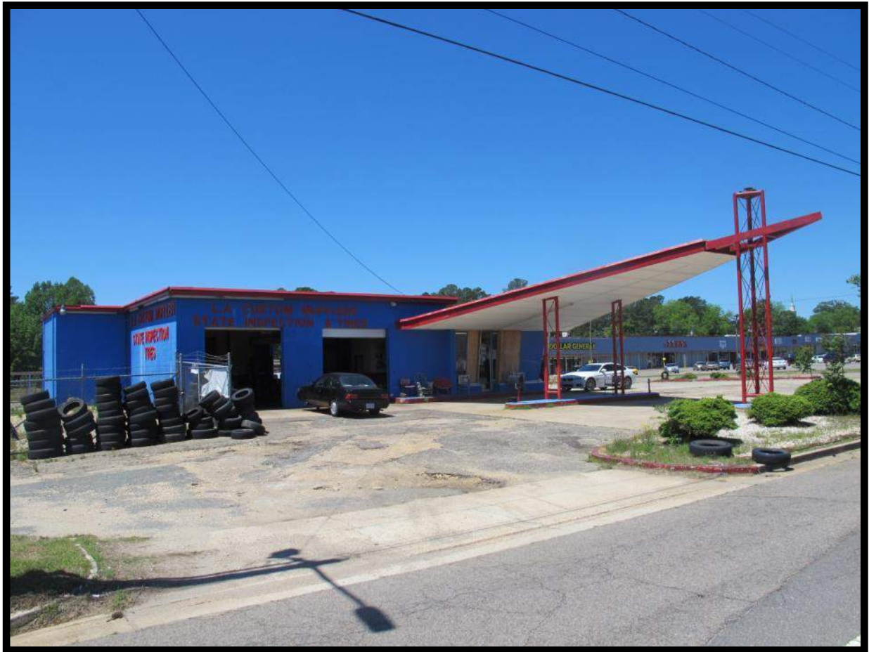
Figure 101: View of a (former) Phillips 66 Service Station at the Corner of Lee Avenue and Judd Street in Sanford, Lee County, North Carolina.
