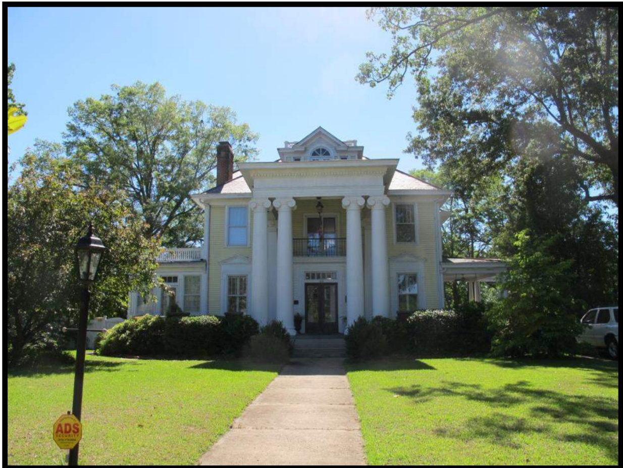
Figure 59: E. L. Gavin House (LE0353), Looking Southwest.
