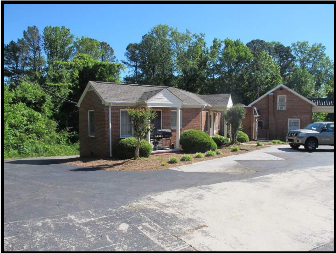
Figure 9: Jefferson Motel, View of Wing Looking North.
