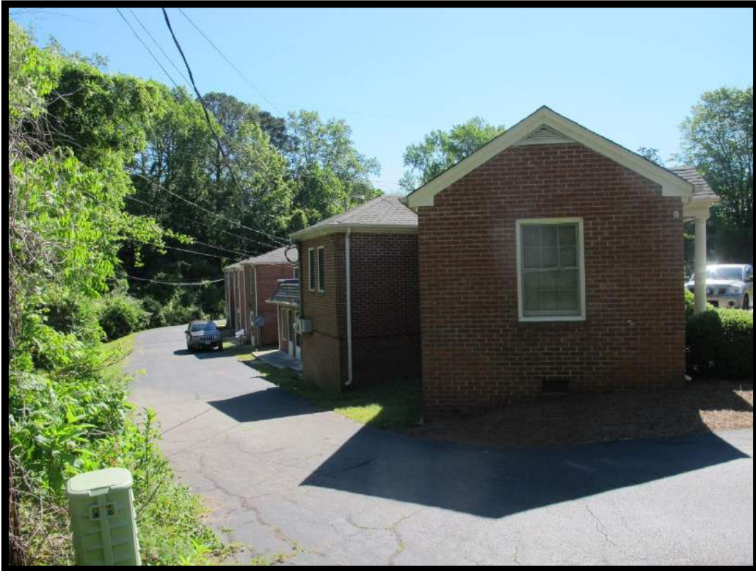
Figure 10: Jefferson Motel, View of Wing Looking Northeast.
