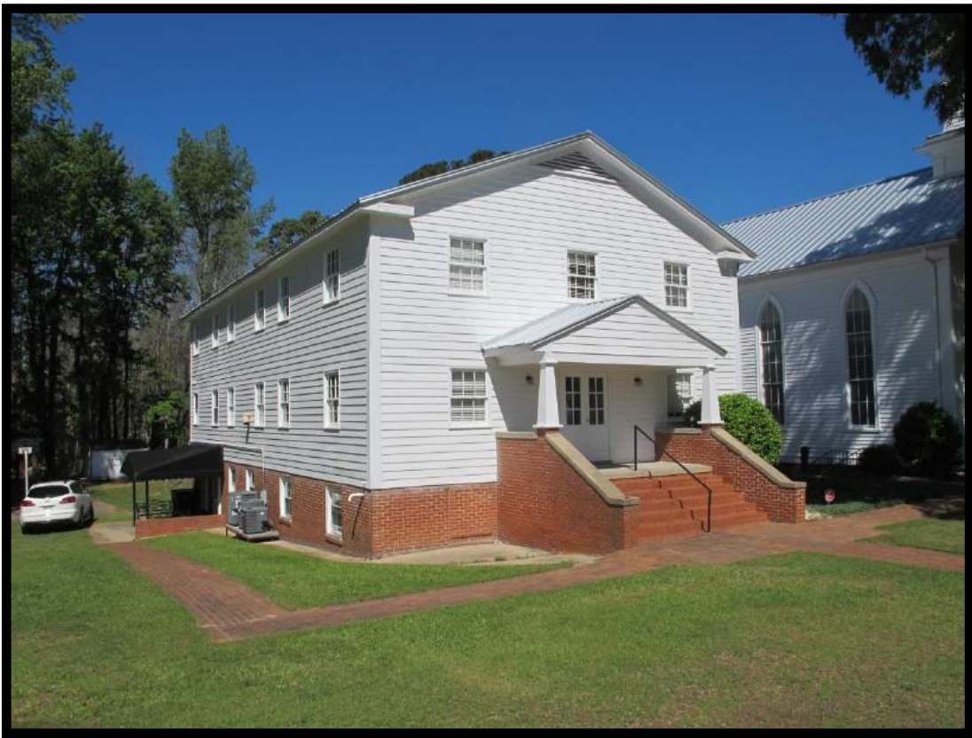
Figure 28: Buffalo Presbyterian Church, Educational Building Looking Northwest.
